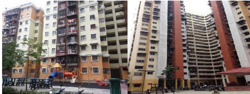
Figure 1. Pantai Dalam development (Source: Google)
